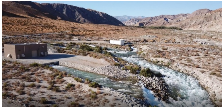
Water from the Colorado River Aqueduct is conveyed through the Whitewater Hydropower Plant and ultimately feeds WWR-GRF.
