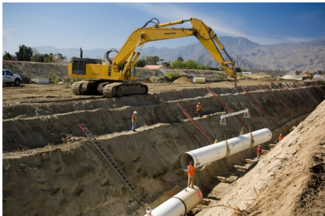
Construction of the Mid-Valley Pipeline in 2009 to deliver Canal water to the Mid-Valley area.
