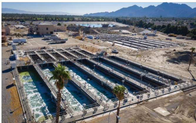
CVWD is planning to connect 29 additional customers to the WRP-10 recycled water distribution system.
