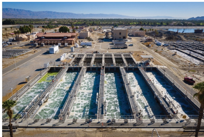
WRP-10 provides recycled water to large irrigation customers in the mid-Valley area.
