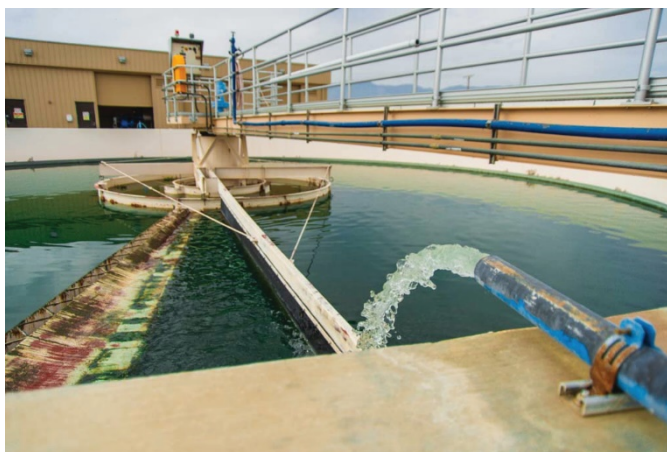
CVWD's WRP-4 has a secondary treatment capacity of 9.9 mgd (11,090 AFY) and has a planned tertiary expansion.
