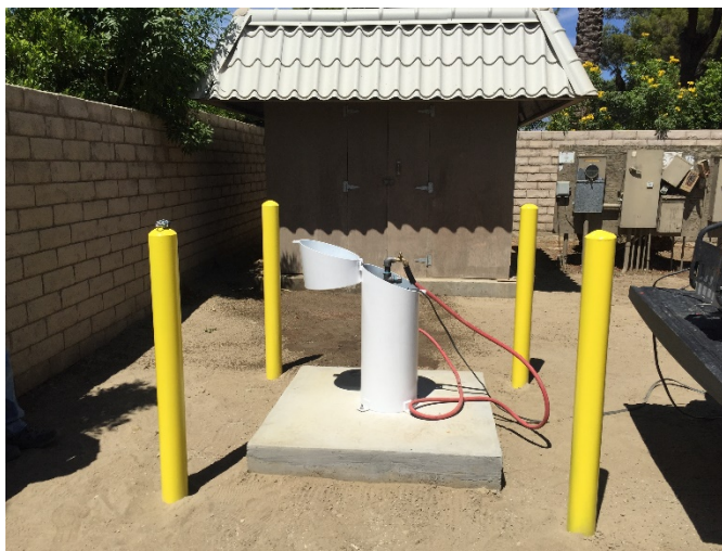
Monitoring well located at PD-GRF.
