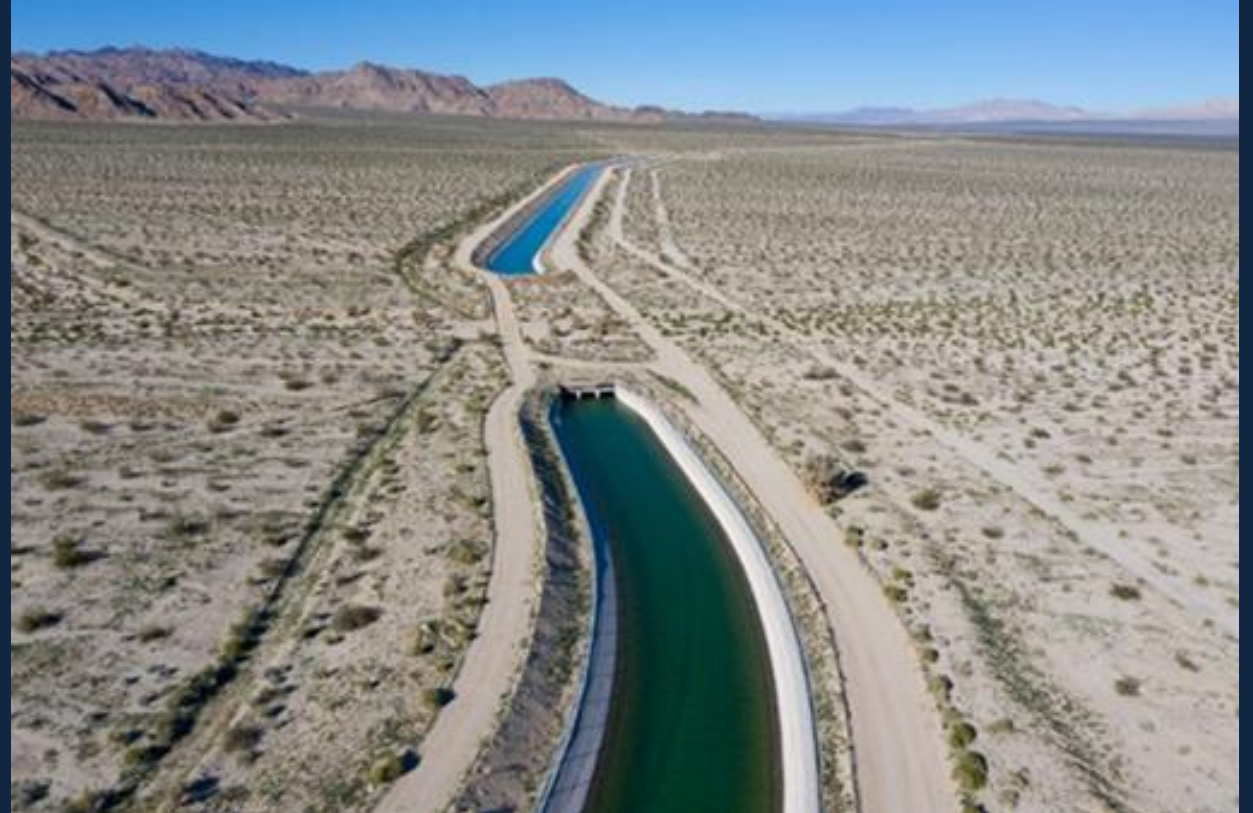
Colorado River Aqueduct
