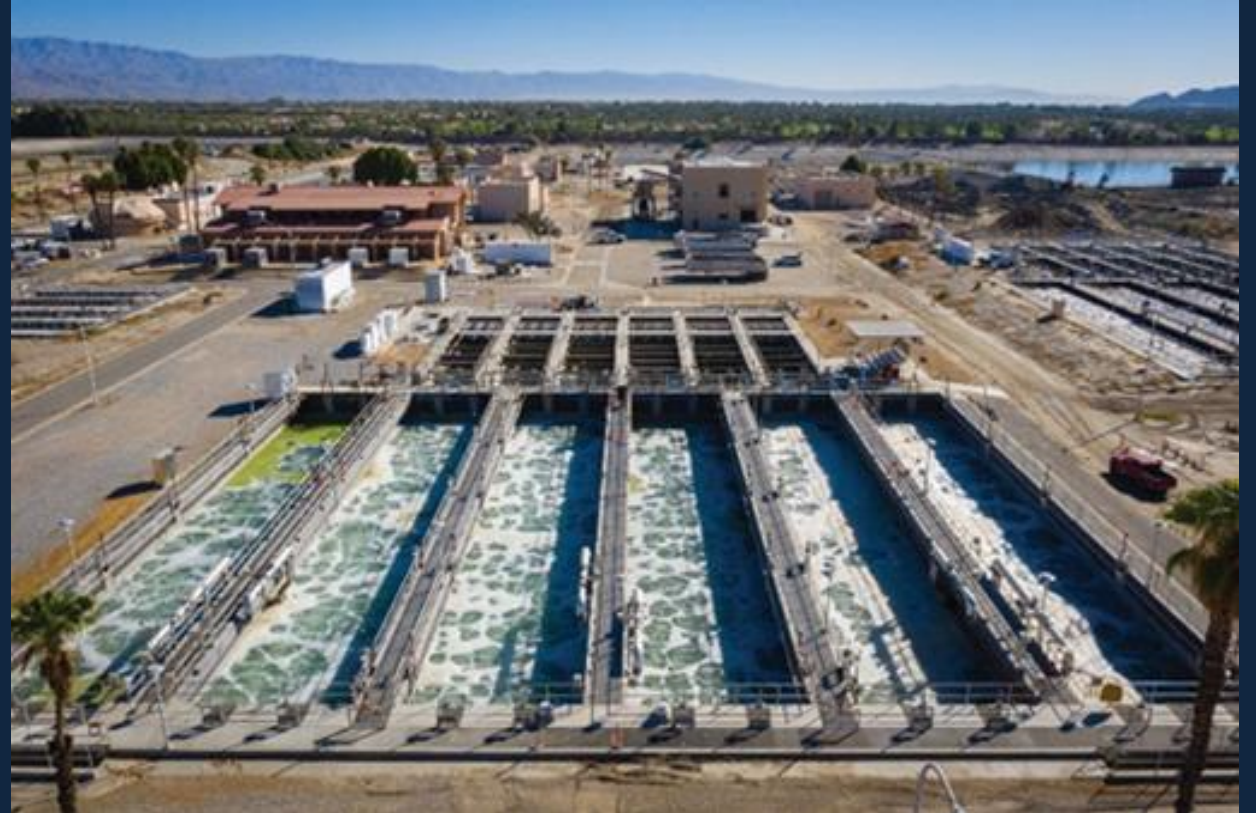
CVWD's Water Reclamation Plant (WRP) No. 10
